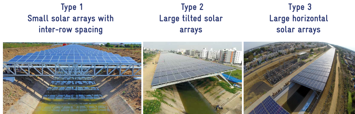
Figure 3: Design configurations for small and medium canals
